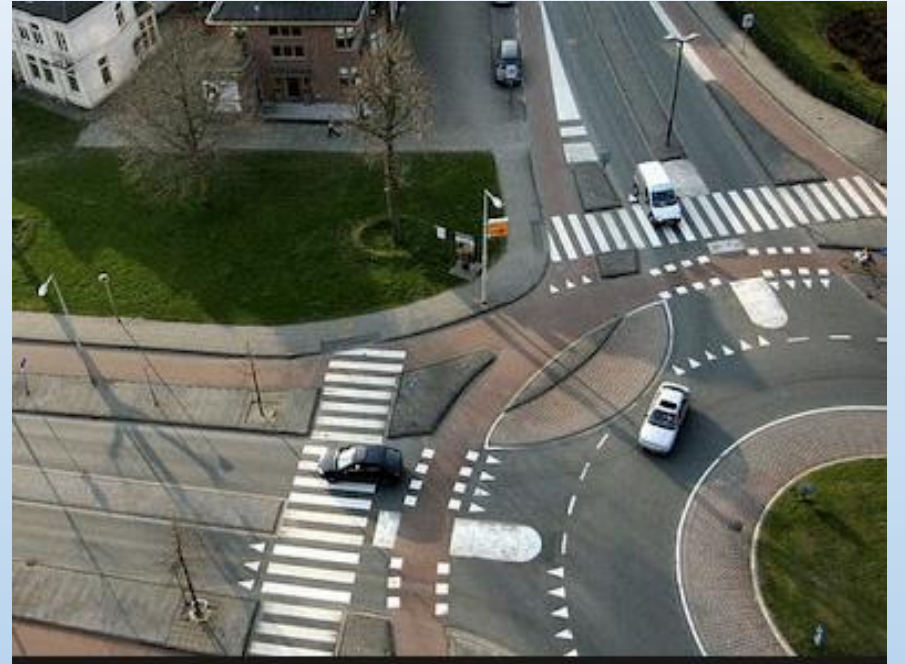
Roundabout in the Netherlands designed with pedestrians, cycles and cars in mind.
