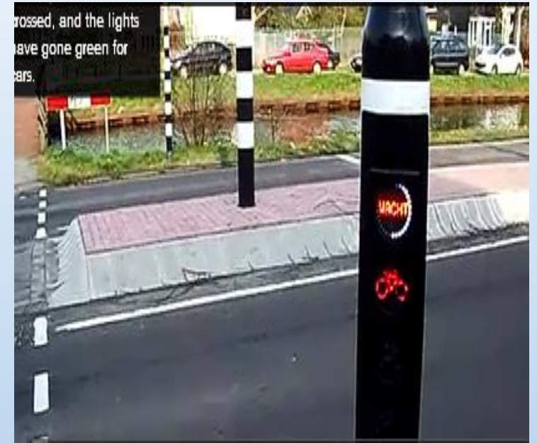
Countdown timer for lights Assen, Netherlands
